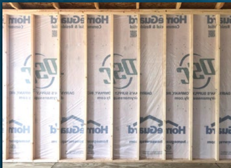
HOUSE WRAP VAPOR BARRIER | P1
